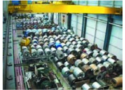
View showing Island Steel's gantry cranes with lifting capabilities of up to 30 Tonne.
